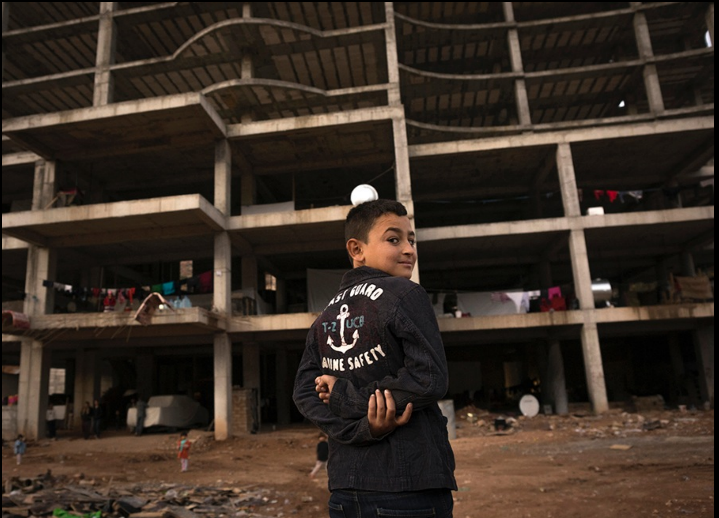
With construction stalled in its early stages, the concrete structure is an inhospitable environment for the 63 Yazidi families, 364 people total, who now call it home.
