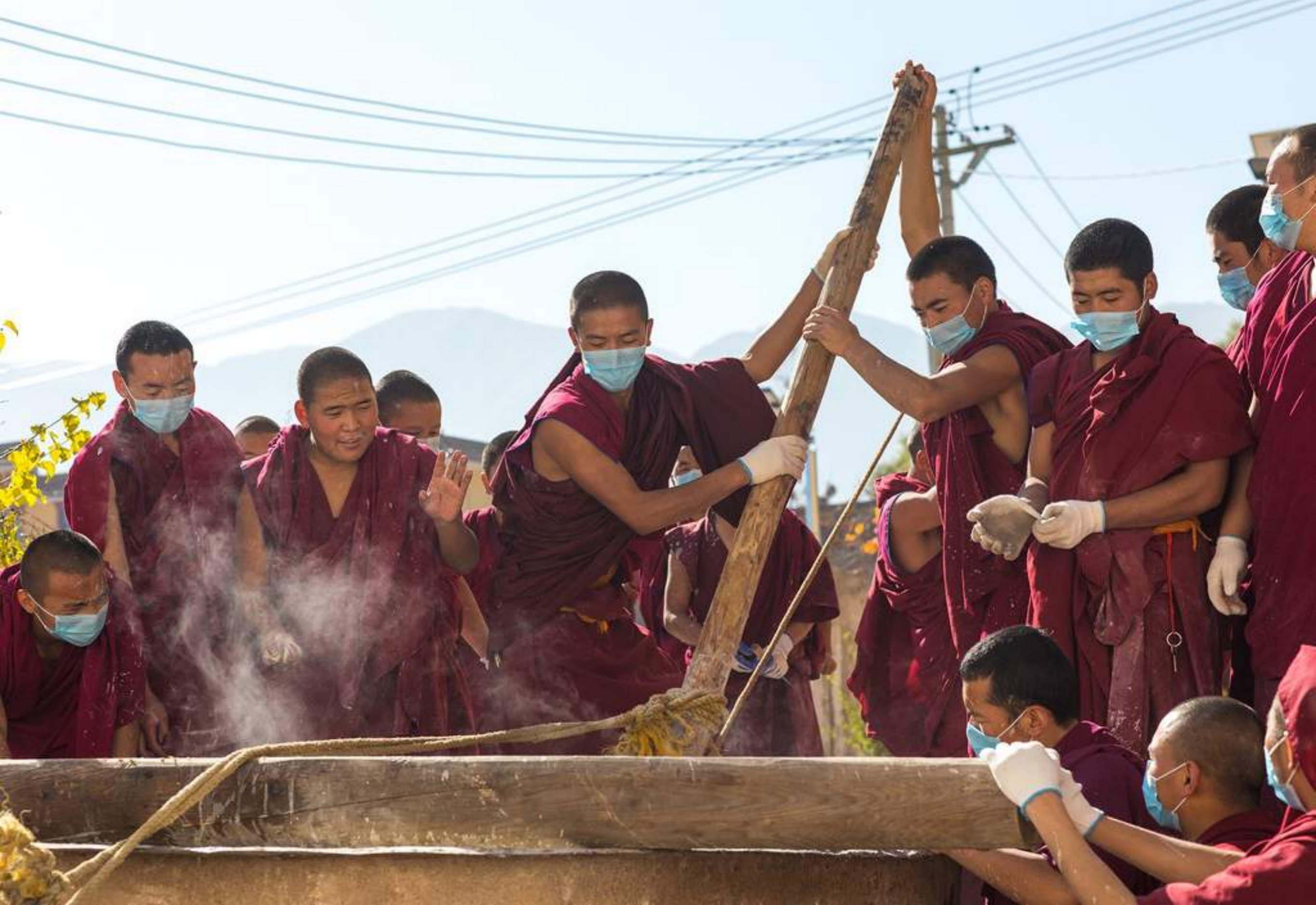
Bags of lime are mixed with hot water in a huge tank. The strongest monks stir the liquid with a giant oar.
