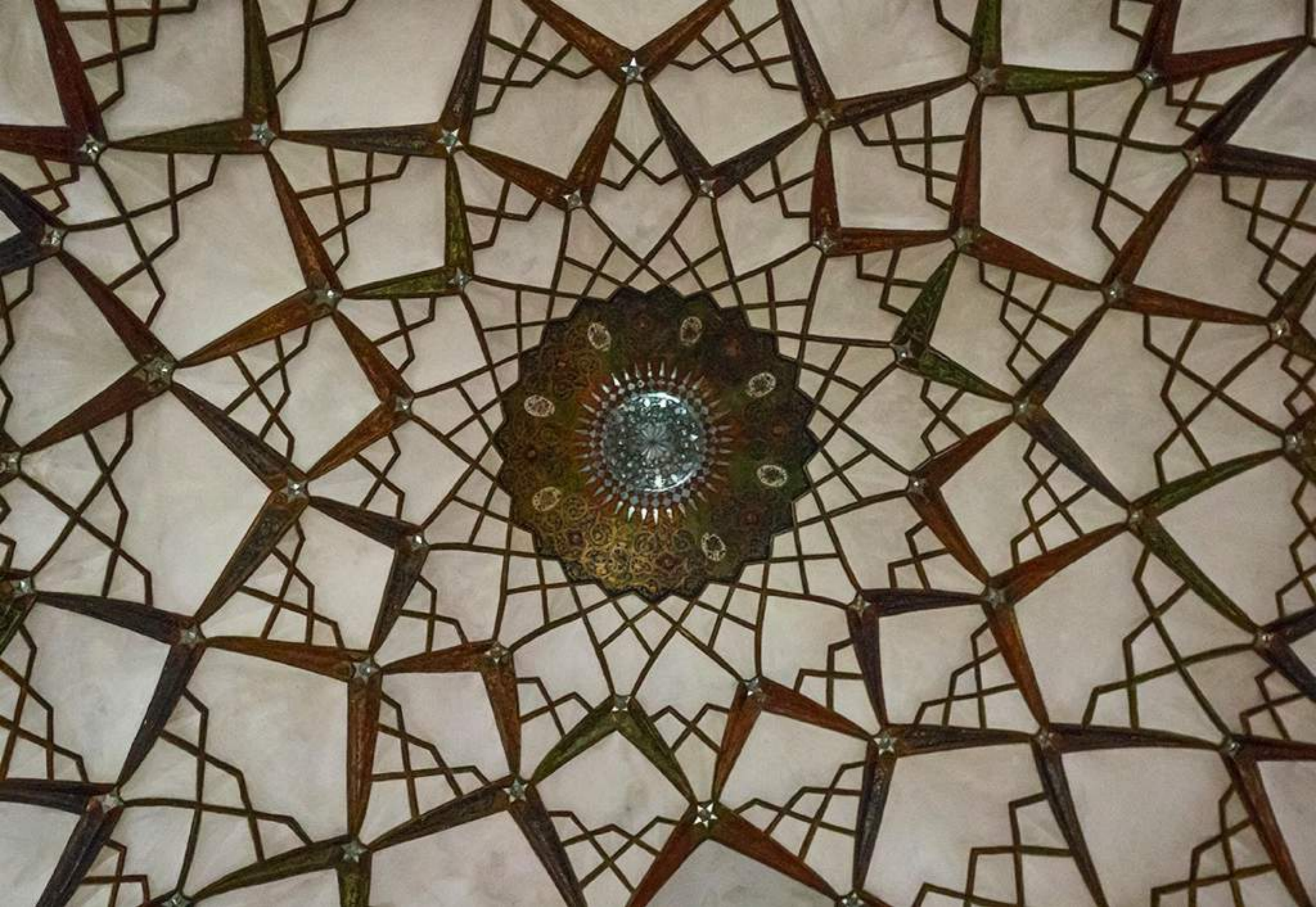
Ceiling In Tabatabaei Historical House built in 1880, Kashan. The picture shows how heavily mathematics and geometry featured into Islamic architecture .
