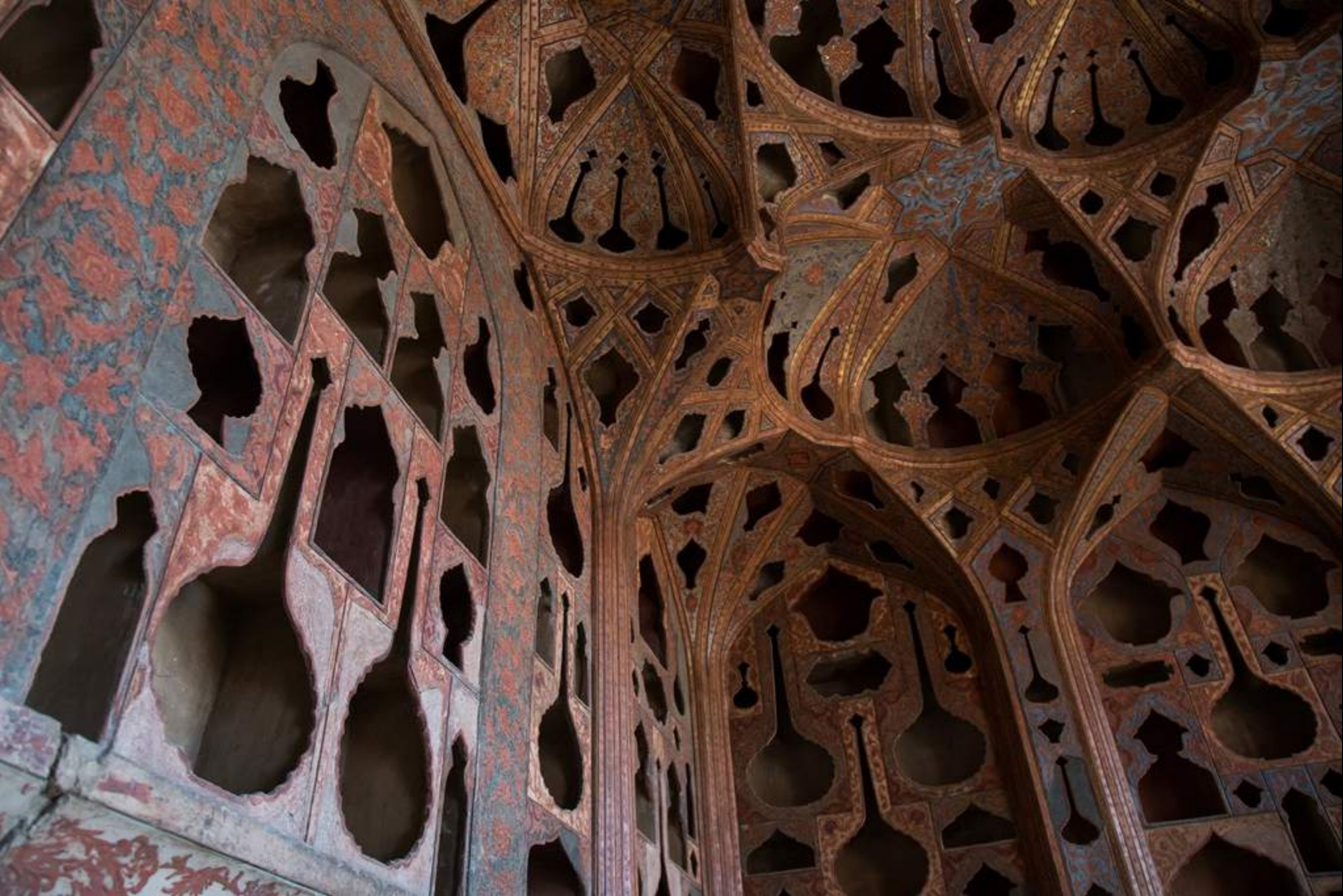
the famous acoustic ceiling in the music room at the top of of ali qapu palace on the 6th floor. The ceiling of the music room has cut out stucco decorations of vases and goblets which served to enhance the sound of music played for the King. isfahan
