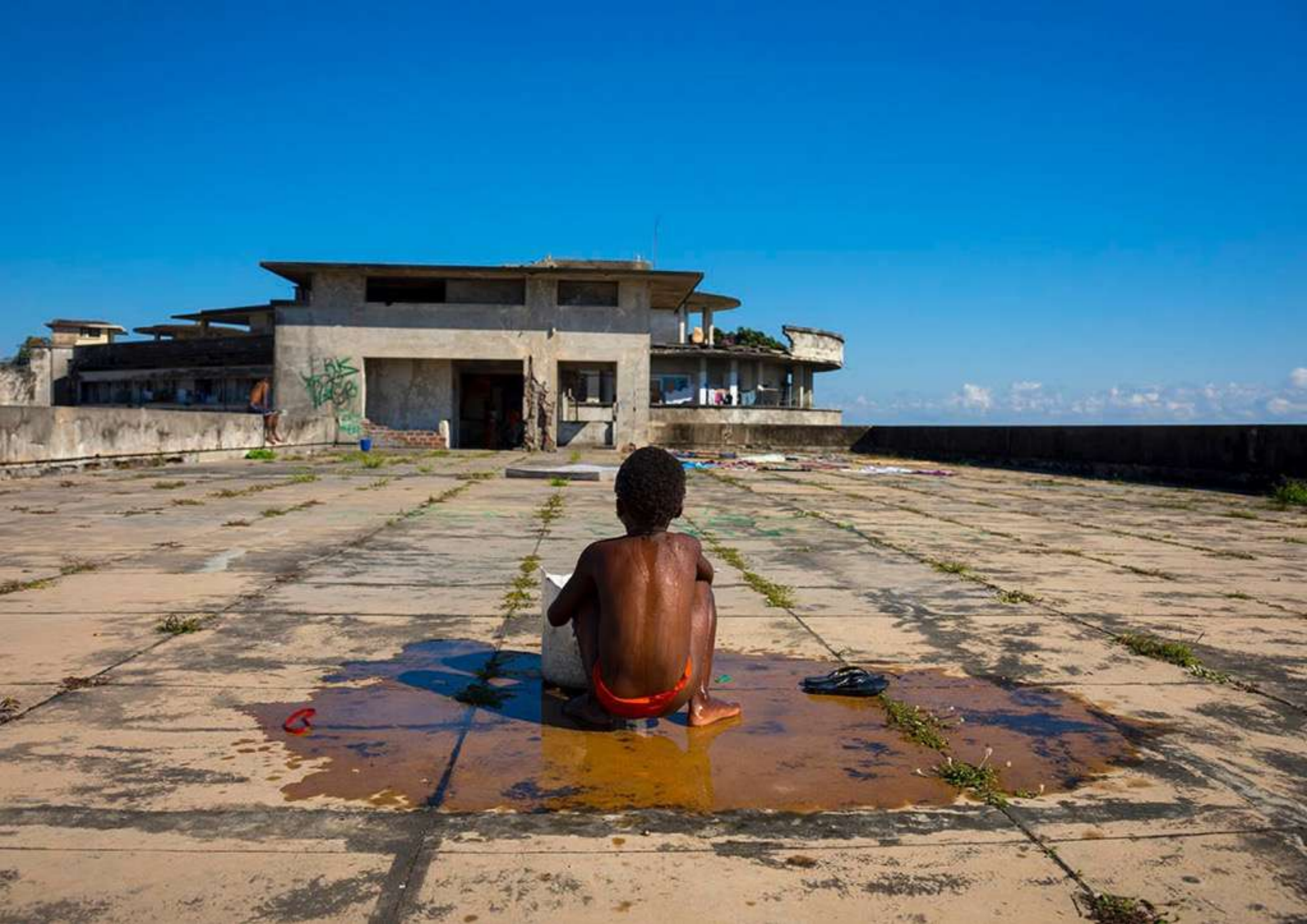
The former helicopter pad has become an open air bathroom...
